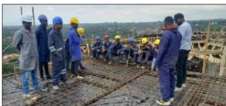
Electrical and electronics students being assessed during an electrical installation attachment
